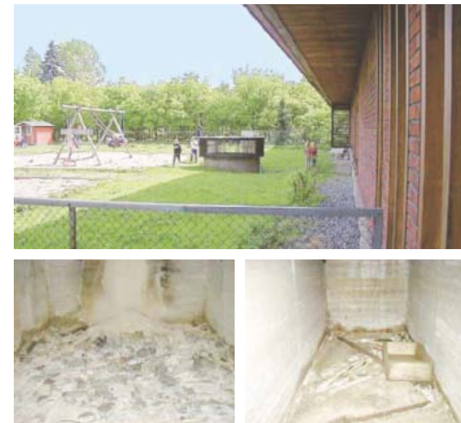
FIGURE 19. Air intakes at easily accessible heights can become waste bins. Abandoned building waste does not improve the situation. Photo: Frode Frydenlund, EPT-SEfAS.
