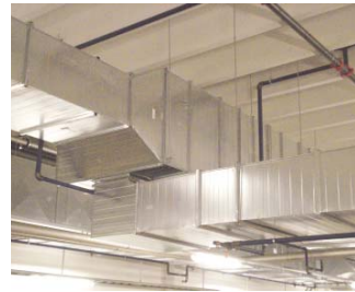
FIGURE 5. Transverse-stiffened duct.
