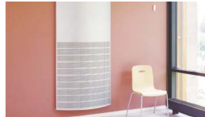
FIGURE 34. A thermally controlled, wall mounted displacement diffuser.
