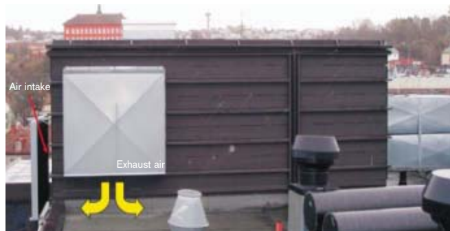
FIGURE 7. Unsuitable location of an outdoor air intake in relation to the exhaust air outlet. There is a great danger of short-circuiting between the two systems and undesirable microbic growth on the surface of the roof – microbes could then find their way into the air intake. Photo: Frode Frydenlund, SINTEF Energy Research, 2007, Trondheim, Norway.
