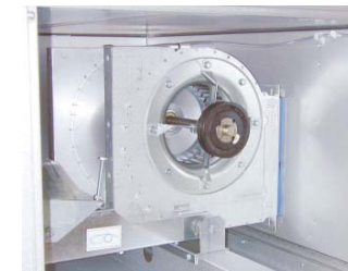
FIGURE 2. A double-inlet radial fan.
