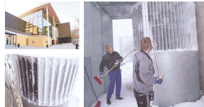
FIGURE 6. De-icing the air intake for a school building in Trondheim, Norway. The school was built in 2004 and the photos taken in early January 2006. Photo: Fredrik Hedeman.
