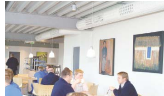
FIGURE 30. Duct diffuser installed in a restaurant.
