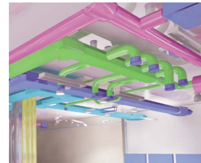
FIGURE 11. Colour-coded ducting.
