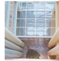
FIGURE 9. Ventilation ducts in two of the atriums at Ramböll's Gothenburg office.
