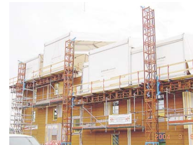
FIGURE 4. Requirements for achieving a good indoor environment can include the provision of weather and moisture protection measures for materials and components, to protect them against moisture and dirt.
