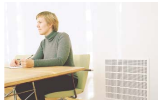
FIGURE 43. A diffuser built into a wall.
